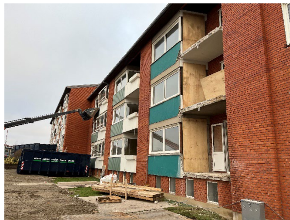
Dec. '24 renovering 8B
